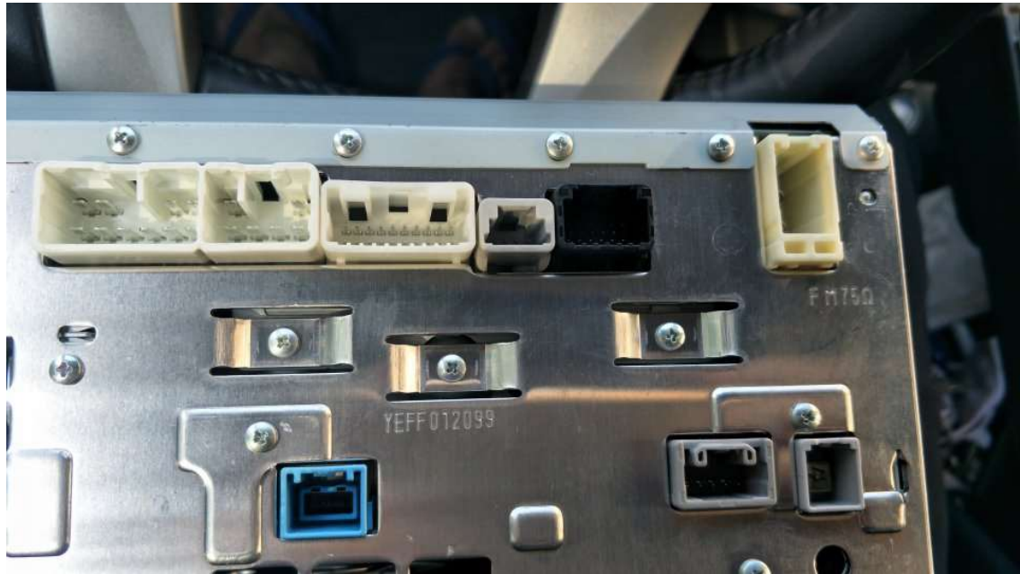
Figure 8 Only the 4 connectors will be needed the 5e with 28 pins is not used.
